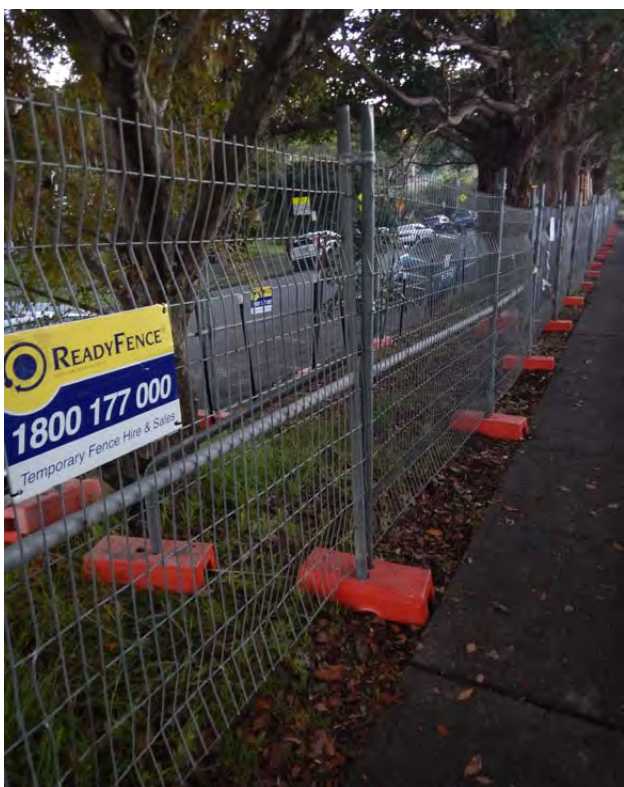
Figure 91- Groups of street trees within a grass strip may also require tree protection fencing installed to protect the trees and the ground surface around them. (Photo: Arterra)
