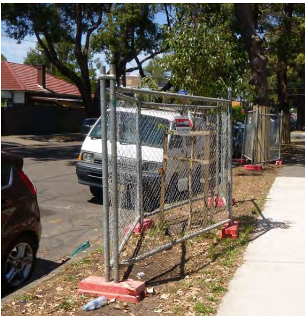
Figure 94- Younger trees that are too small to apply trunk protection shall be fenced as above to protect the roots, foliage and trunk during construction periods. (Photo: Arterra)
