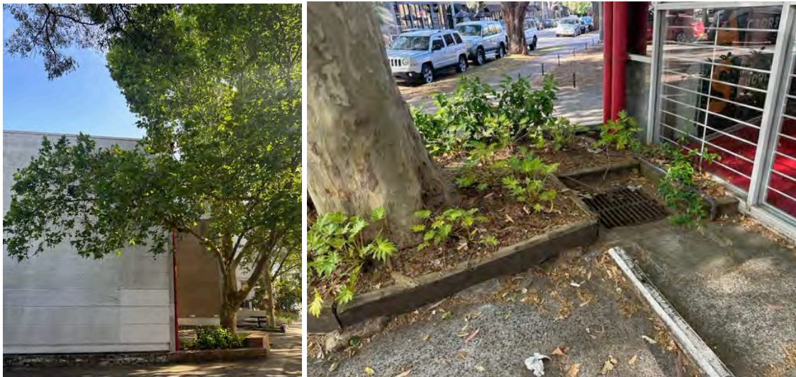
Figures 46 & 47: The proximity of Tree 4 to the existing building edge (Left) and the slab and drain between the trunk and the building(Right). (Source: Austin 2 nd November 2023)
