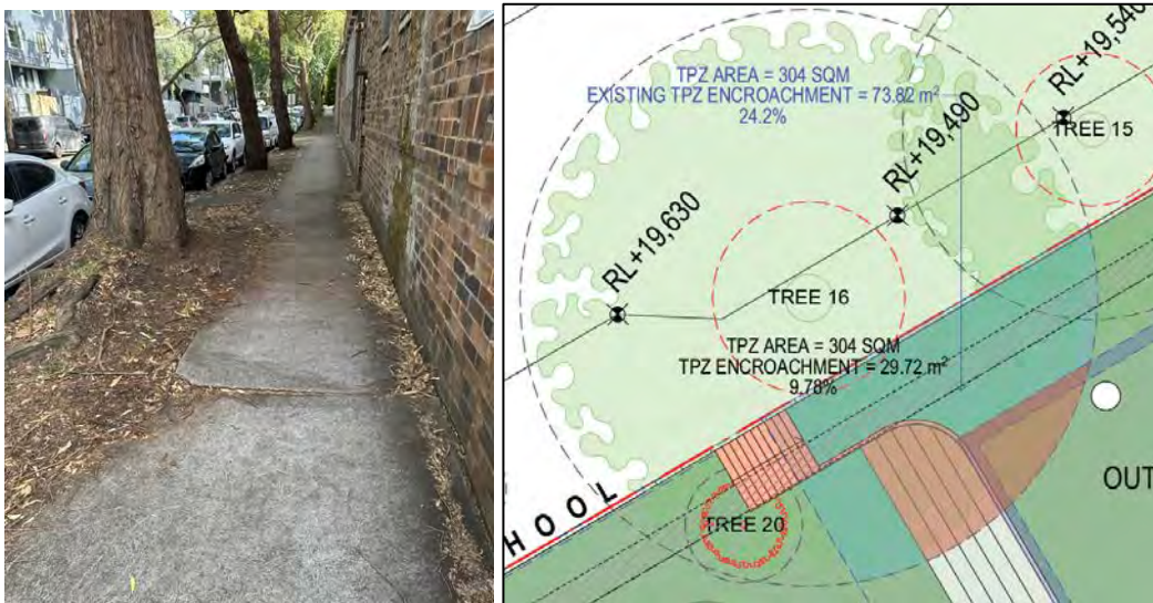
Figures 80 & 81: The proximity of Tree 16 to the existing building edge depicting the lifted paving (Left - Source: Austin 2 nd November 2023) and the floor plan depicting the existing building in the blue hatched line with the proposed building TPZ encroachments shown in pink, batter in blue and scaffold from level 1 and above shown in hatch (Source: General Floor Plan, by Plus Architects, drawing number PLA-PP -1000 dated 15/1/2024). See appendix for larger plans.
