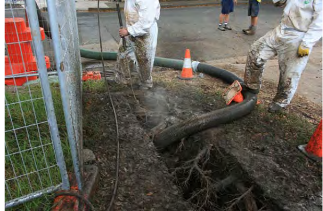
Figure 95- Hand excavation or other non-destructive methods such as water jetting and vacuum extraction to excavate around tree roots. (Photo: Arterra)
